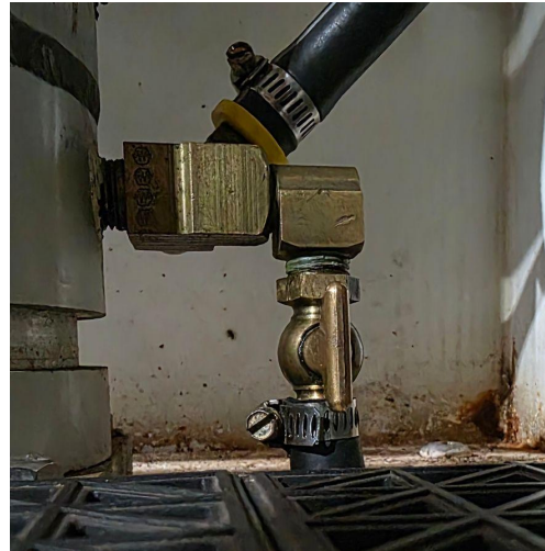
Figure 5.2 - Option B Open the mast valve.
